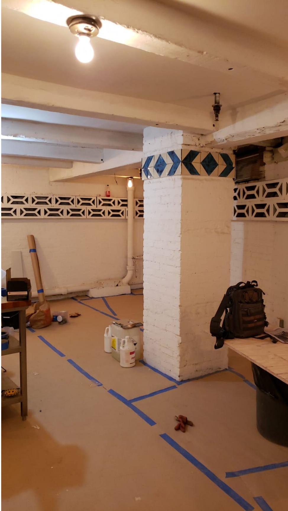
DINING AREA IN RENOVATION
