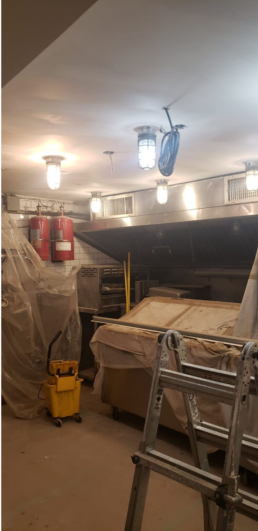
KITCHEN AREA IN RENOVATION
